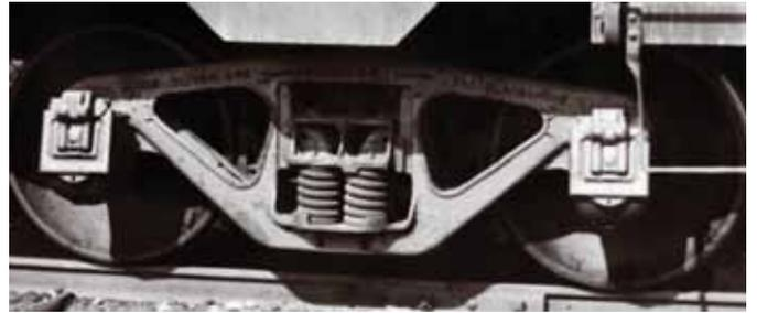
**Fig. 8 BARBER S-2 TRUCK.** The Barber Stabilized truck design was among the most commonly used types of freight car trucks through the end of the solid-bearing-truck era.
